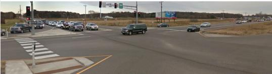
The US 169 Rural Safety and Mobility Interchange Project will reconstruct approximately one mile of US Highway 169, an existing Principal Arterial roadway, from a rural four-lane undivided highway to a four-lane divided expressway and construct a grade-separated interchange at County Road (CR) 4.
